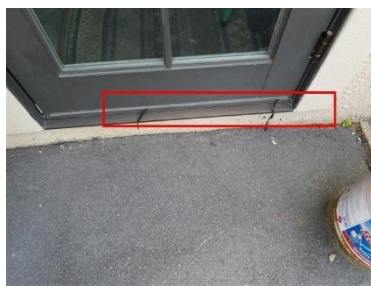
2.1 Item 2 (Picture) garage
