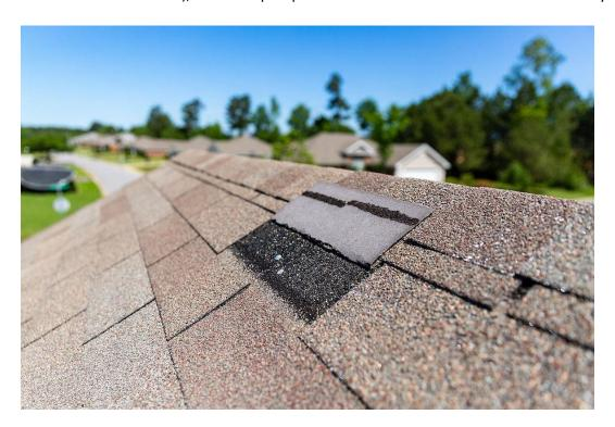
The inspection image of the roof shows a shingle tab that lifted up in the wind and cracked in half. This is a roof defect that happened after a home inspection was performed. This problem is not the responsibility of the home inspector, but of the homeowner. And it's likely that the homeowner wasn't aware of the problem.
